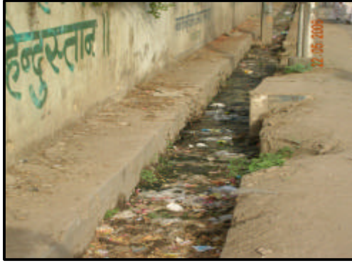
Flow of sewage and disposal of solid wastes in drains. Silting and blockage of secondary
